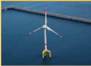
Tri-pile foundations
