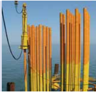
MHU 270T – conductors
