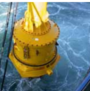
"little bubble curtain" surrounding pile
