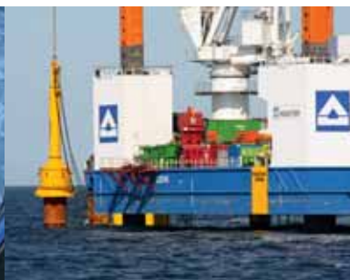
MHU 500T driving tripod piles
