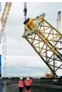
Jacket to be installed onto 4 piles
