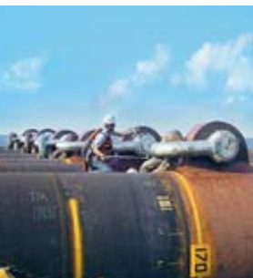
Piles with pad eye
