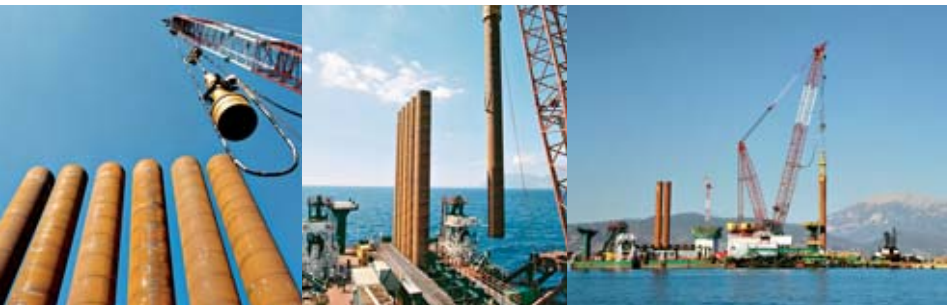
Hammer above waiting piles
