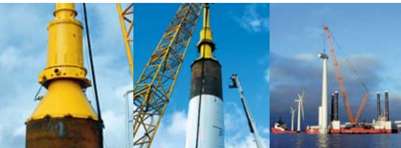
MENCK MHU 600B with 4.5 m pile adaptor
