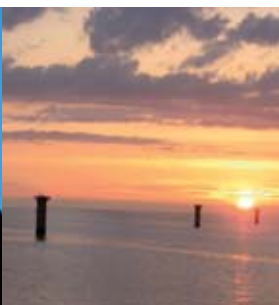
Monopiles waiting for windmills
