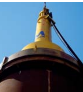
MENCK MHU 800S with 5.2 m pile sleeve
