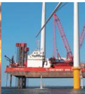
Installation of windmill towers on monopiles
