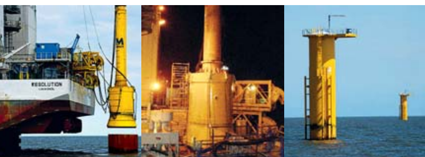
MENCK MHU 1900S being removed from pile
