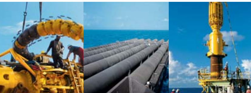
Assembly umbilical to hammer
