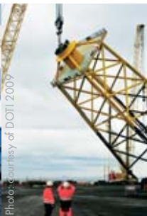
Jacket to be installed onto 4 piles
