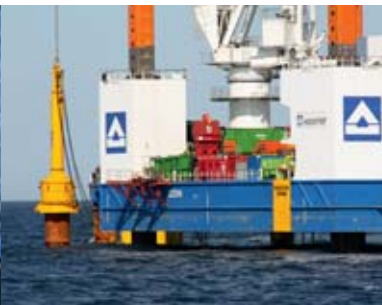
MHU 500T driving tripod piles
